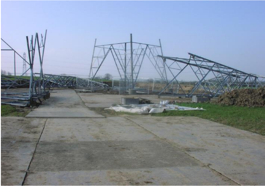
Photo B-3: Pylon Construction Site Showing Partial Assembly at Ground Level
