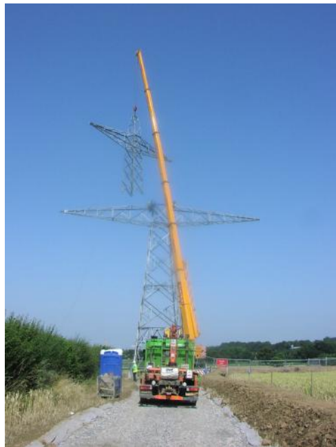
Photo B-4: Pylon 'Peak' being Lifted into Place
