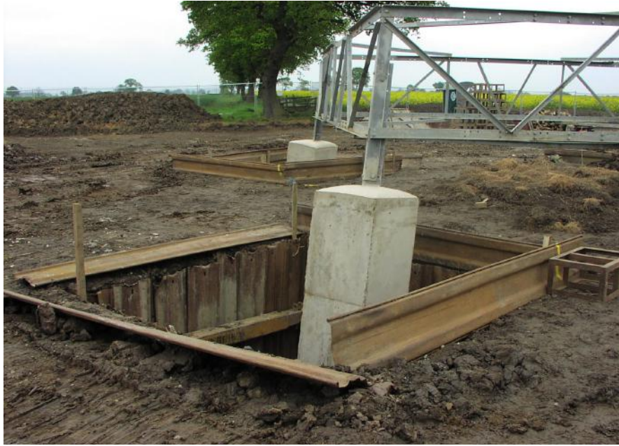
Photo B-2: Steel Foundations for Pylon Legs
