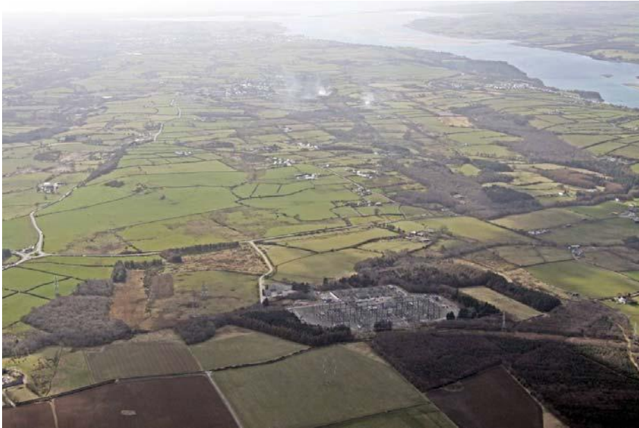
Photo Number 37. View of Pentir Substation looking south west toward Bethel. (11479-87).
