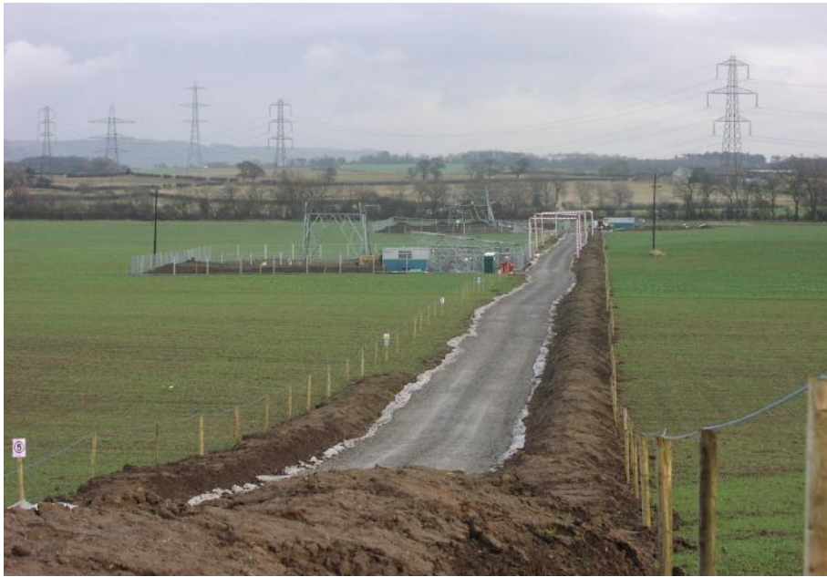
Photo B-1: Temporary Stone Access Track with Demarcated Pylon Construction Area
