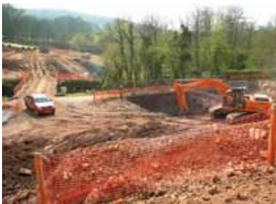
Before Construction of one of two new gas pipelines through the south west.
