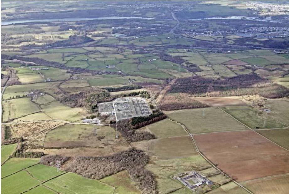
Photo Number 33. View of Pentir Substation looking north west to Vaynol and Britannia Bridge. (11479-95).
