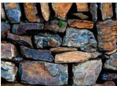
A reinstatement to a road crossing on the route of The South West Reinforcement Project. The breach was repaired using traditional Devon Banks methods.
