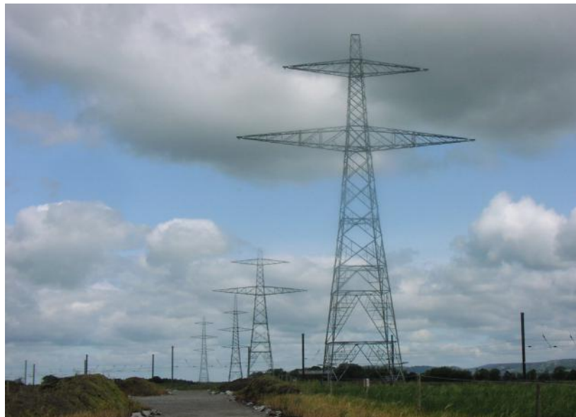
Photo B-5: A Line of Pylons Waiting to be Strung
